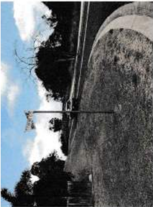
PHOTO 17 - Example of insufficient clear sight distance when regulated or higher speed (as is frequent) is encountered
