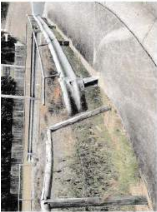
PHOTO 22 - Damage to armco safety rail and adjacent safety handrail - unrepaired 4 months after accident due to speed.
