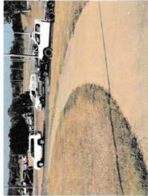
PHOTOS 7 & 8 - As queuing builds, driver frustration builds with vehicles driving across the footpath in order to turn left at the roundabout - poor traffic movement design - road intersection / school entrance juxtaposition.
