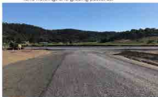
Figure 7 - View west from Mulambin Road towards the Tanby Road intersection under construction
