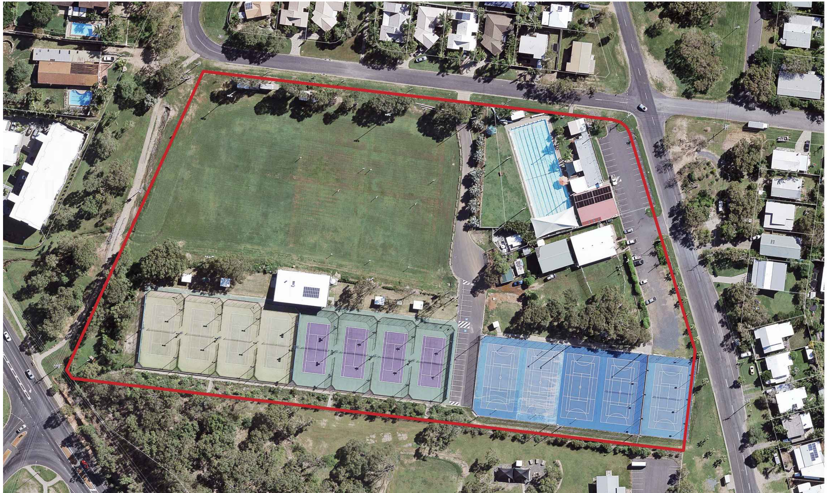
Figure 1: Cooe Bay Sports Complex
