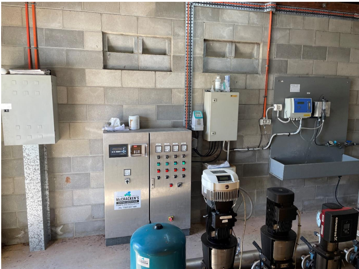
Pacific Heights Booster Pump station – existing switchboard and pumpset to be replaced.
