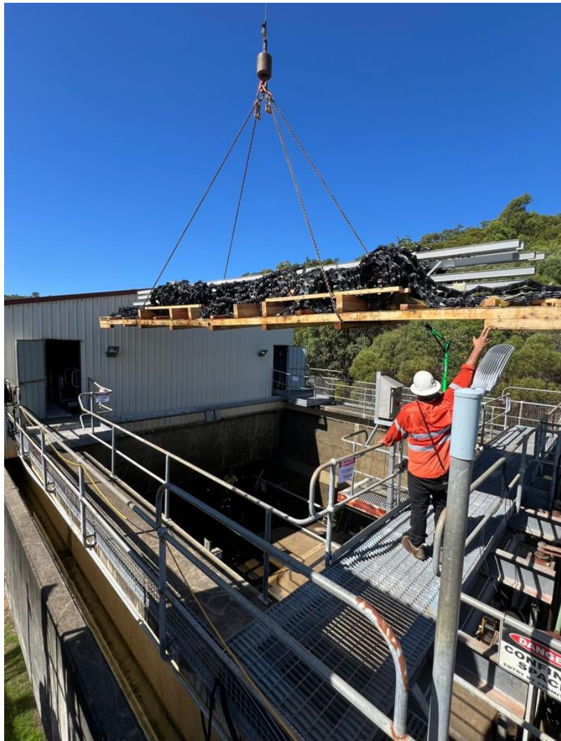
Woodbury WTP Clarifier Scraper Replacement
