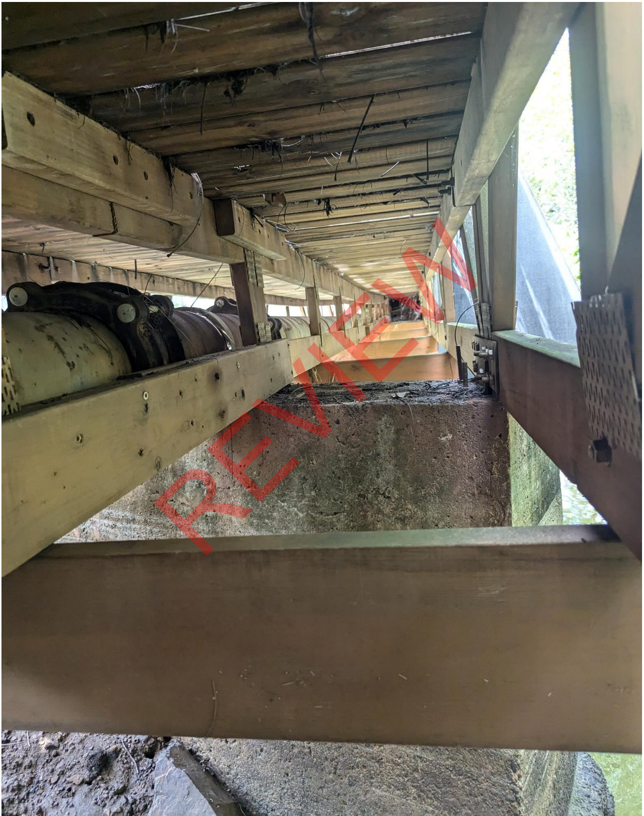
Photograph 3: View of the underside of the bridge deck. Note the existing water pipe does not appear to be supported by the timber bridge. Note the nail plate on the central right of photo is not fully engaged into the truss web members.
