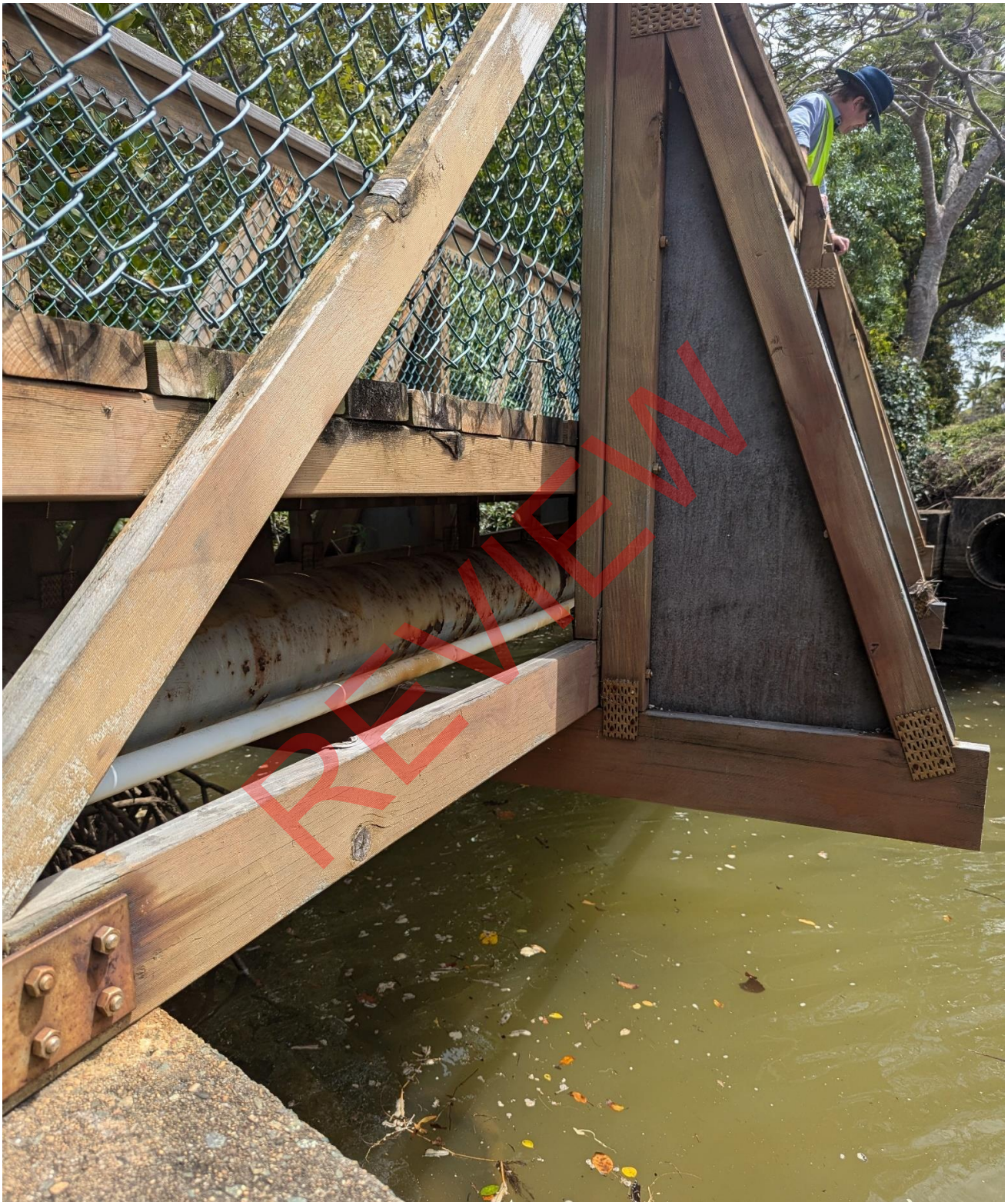
Photograph 2: Underslung bearers with truss top chord lateral buckling restraint outriggers.
