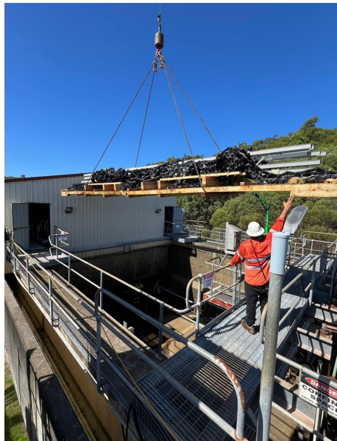
Woodbury WTP Clarifier Scraper Replacement
