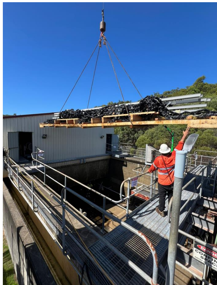
Woodbury WTP Clarifier Scraper Replacement
