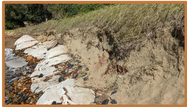
**Figure 51: Erosion occurring above groyne sandbags**
