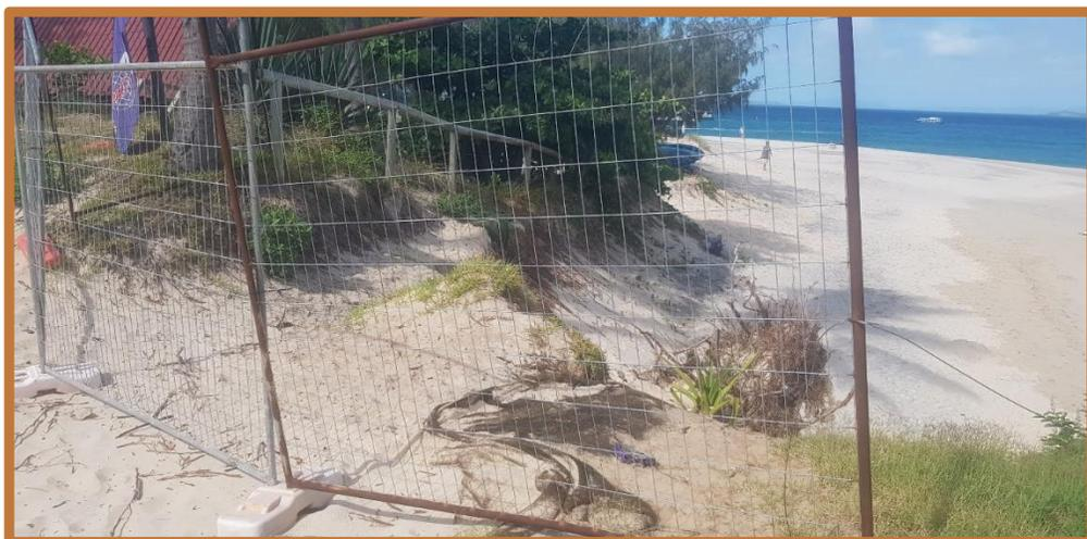
**Figure 59: Erosion between Putney and Fisherman's Beach behind the seawall**
