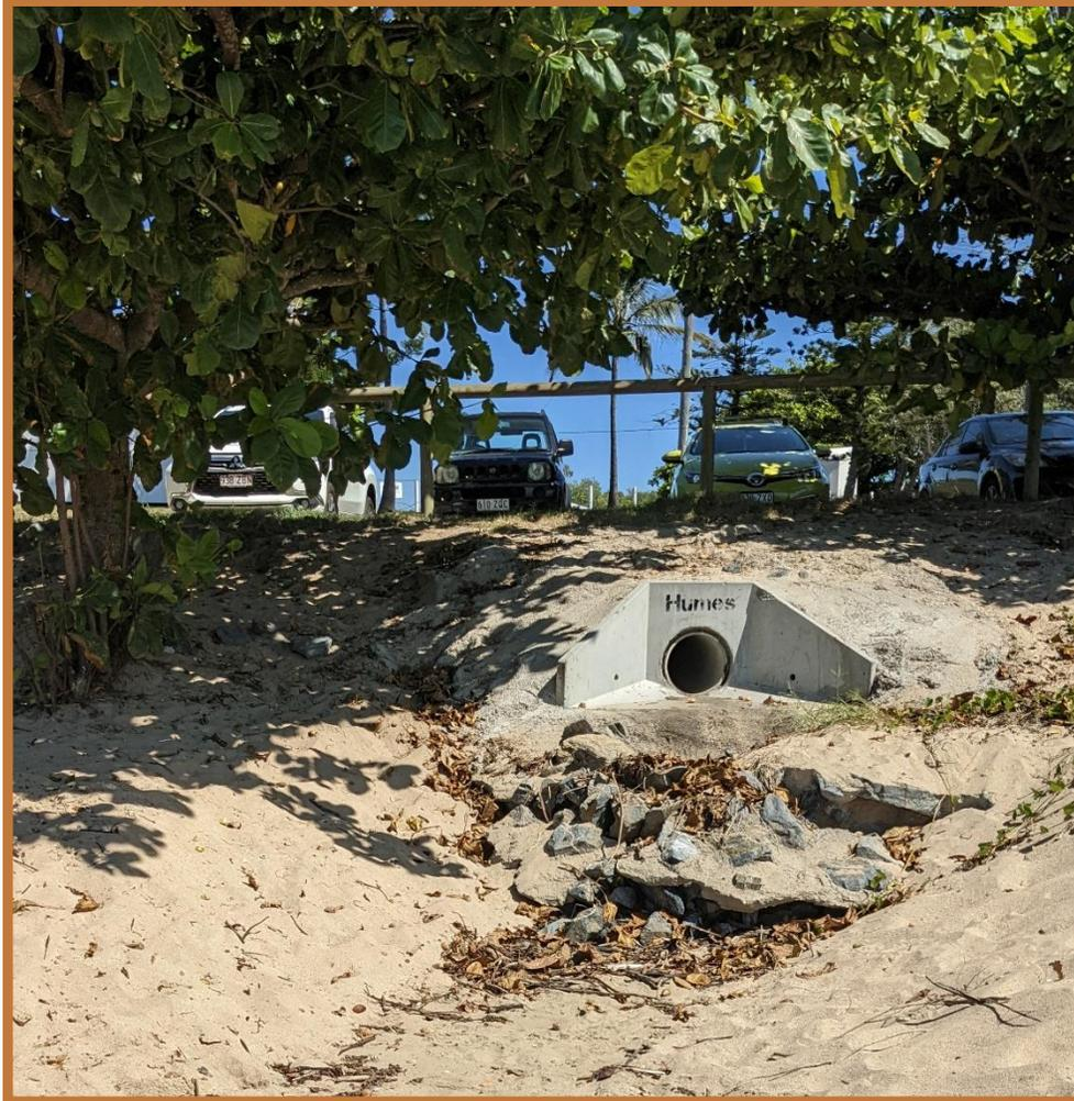
**Figure 28: Channelling at drain located at Cooee Bay**
