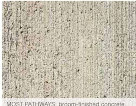
MOST PATHWAYS: broom-finished concrete, utilising colours to indicate wayfinding and pathways connecting key site attractions/uses
