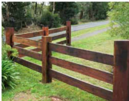
DECORATIVE FENCE Beach Access Locations Hardwood Timber Post and Rail Fence
