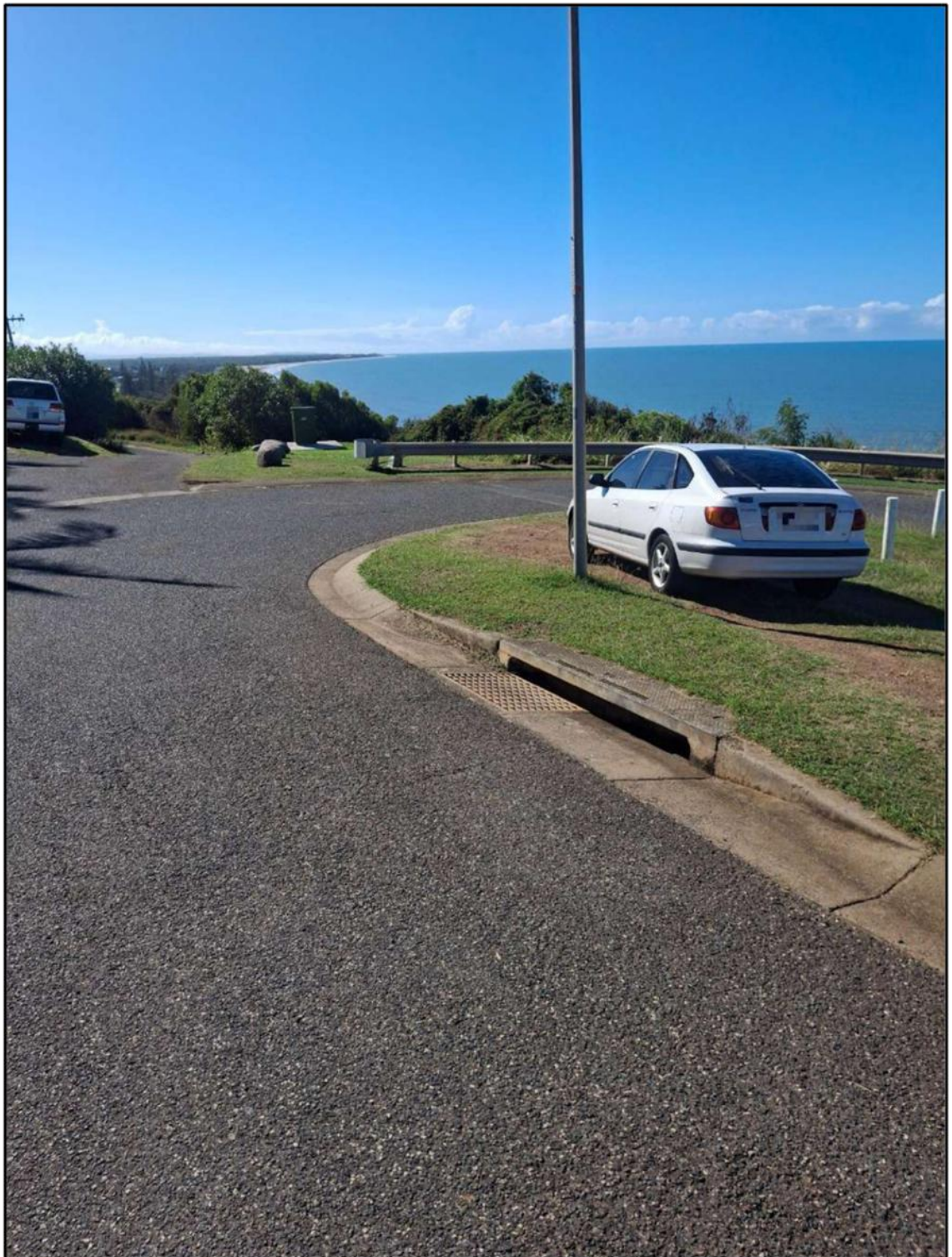
Figure 4 Tight Radius Bend on Northern Entrance to Carpark
