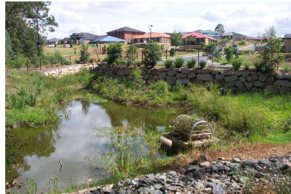
Ill-considered development layout following by poor design by engineers. The result is problematic stormwater management infrastructure which are considered toxic assets by park planners and asset managers
