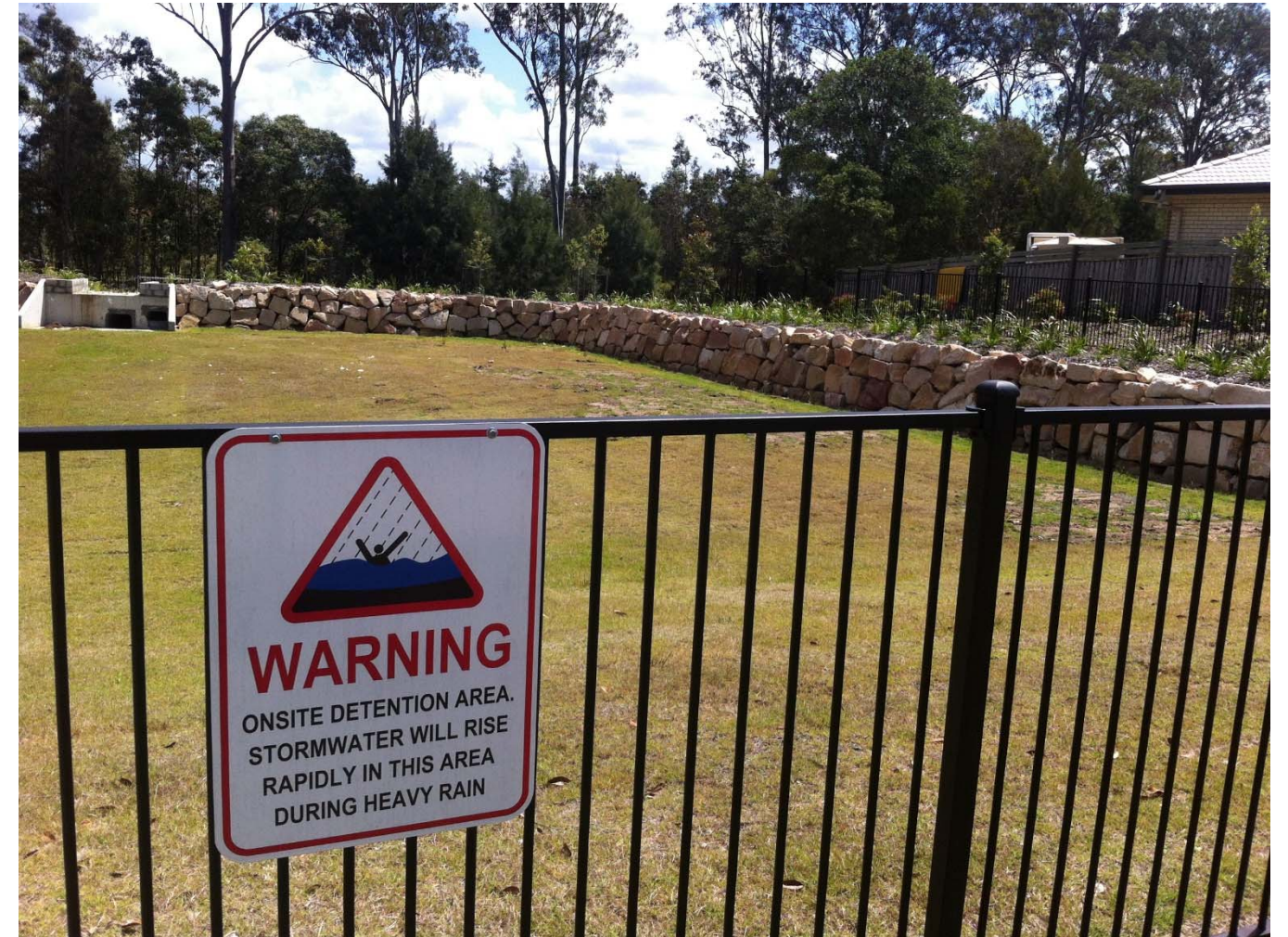
Photo of the Local Park Micro Scale Case Study – Existing stormwater management system not collocated with Local Park and poorly integrated with surroundings resulting in walls and fences. Expensive capital cost and difficult to maintain.
