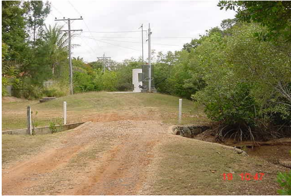
Plate 6 – Lyndall St Pump Station (Note Mangroves on two sides)
