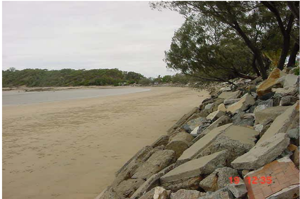
Plate 1 – Seawall at low tide, south end at Keppel Sands beach.
