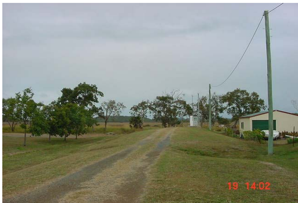
Plate 5 – Rosslyn Street Pump station (Note salt pan in background)
