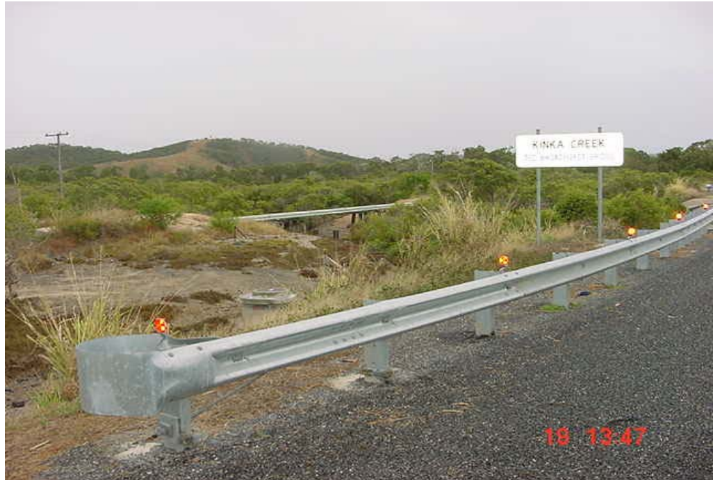
Plate 7 – Water supply across Kinka Creek.
